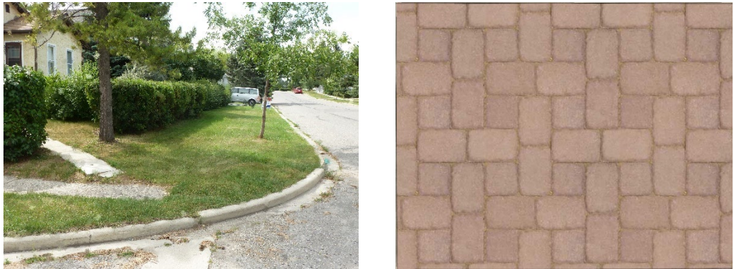
Figure 3.2.1: an illustrative example of soft (left) and hard (right) landscaping as per 3.2(1)(2) of this section.
